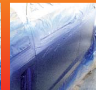
Over the top of the silver goes the Cobalt Blue Kandy, which is making up most of the car's lower half
